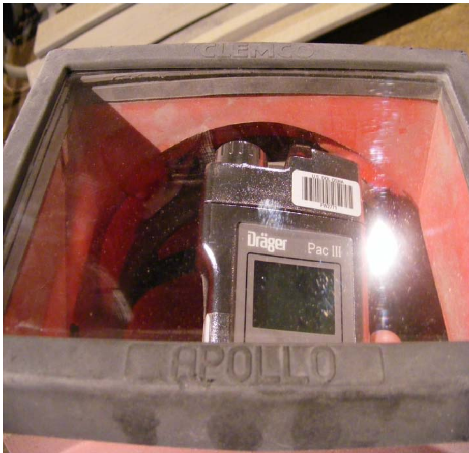
This abrasive blasting hood is being fed with air that is contaminated with carbon monoxide. The source of the air is not from outside, the air is not being passed through a sorbent bed and there is no carbon monoxide monitor or alarm. The meter shows 51 PPM and the limit is 10 PPM.
